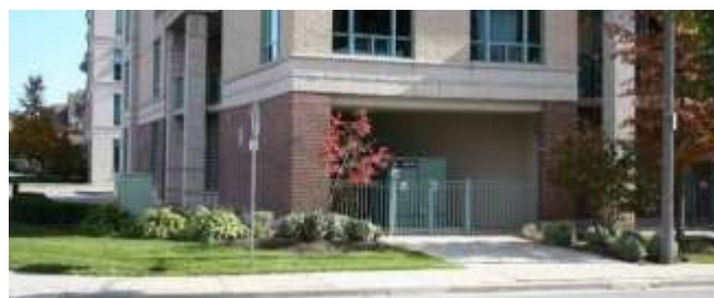
Hydro transformers are effectively screen by integrating in internal bays rather than outdoor locations (Toronto).
